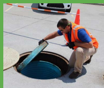
Inspecting a containment sump
